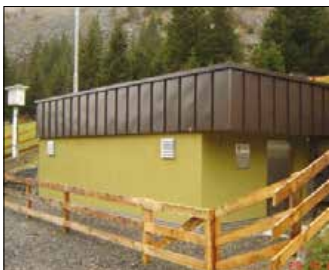
Pumpstation Neurur (Foto: Venier)
